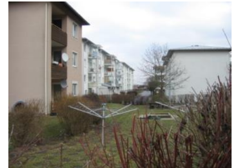
Apartments on local distribution grid
