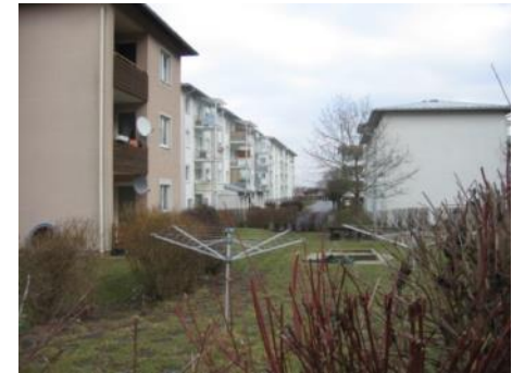
Apartments on local distribution grid
