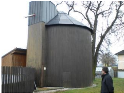
Farm-based AD plant
